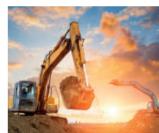
Heavy Road Construction
